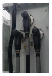
Step 2 Disconnect all communication and power cables between the transformer and the power distribution cabinet and the communication box. Do not leave the removed cables inside the transformer room.
