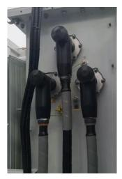
**Step 2** Connect all communication and power cables between the transformer and the power distribution cabinet and the communication box.
