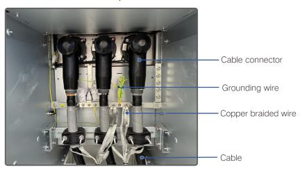
**Step 2** Remove the cables, copper braided wires, and grounding wire inside the RMU (Instructions are given with cables connecting the RMU to the transformer taken as an example; the removal of other cables is similar).
