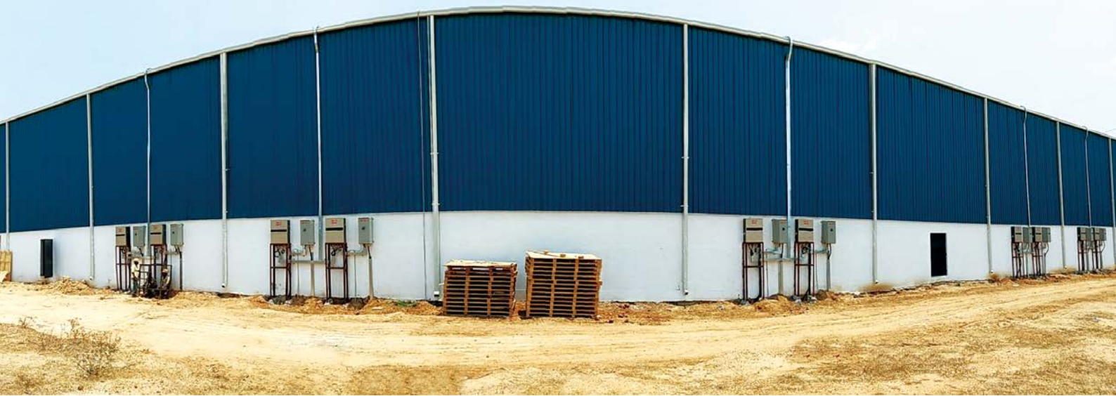
2 MW PV Plant India
