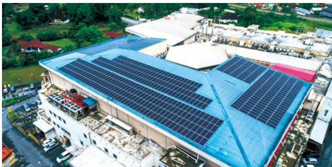
227 kW PV Plant Malaysia
